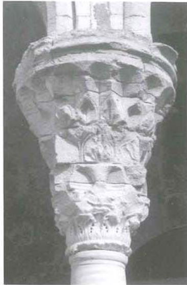
50 and 51 Columns of west porch at Hagia Sophia. In both cases the muqarnas impost blocks were designed to accommodate the different re-used early Christian capitals
